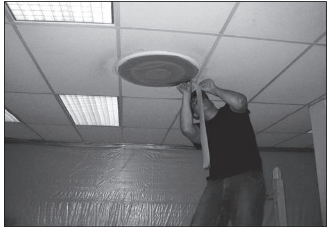
Sealing the ventilation system
