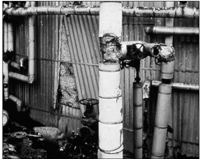
Loose fill insulation
