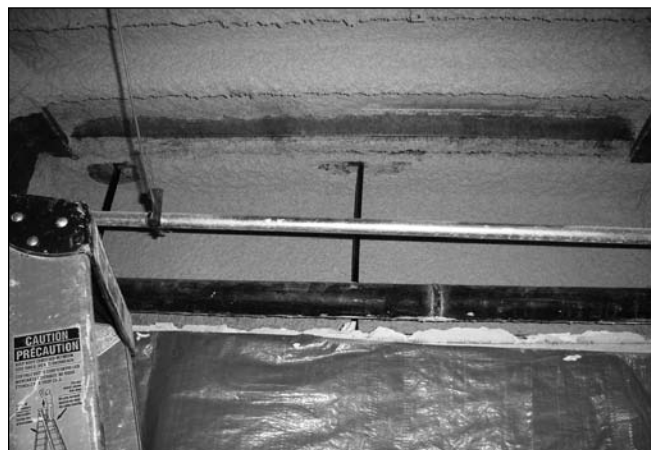
Sprayed-on fireproofing
