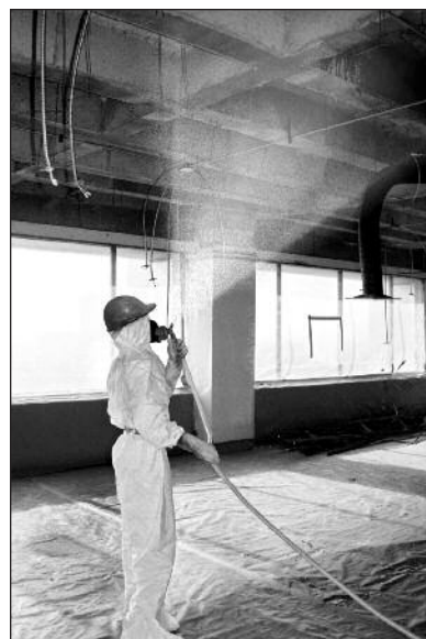
Spraying Asbestos Ceiling Material with Amended Water Before Wet Removal
