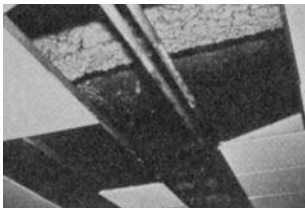
Suspended Ceiling Concealing Fireproofing
